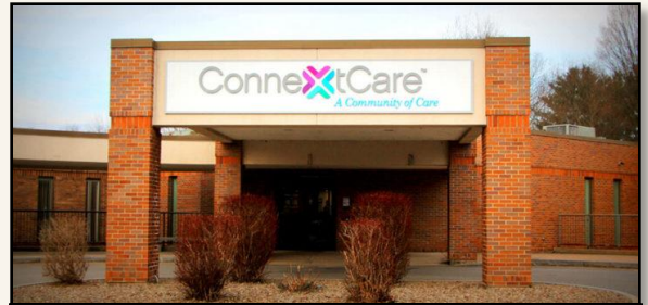
ConnexCare on Delano Street
