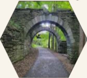
Railroad Arches located on the walking trail
