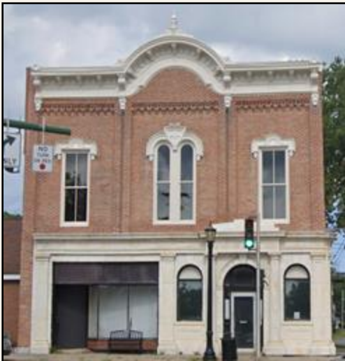
Peoples National Bank Building
